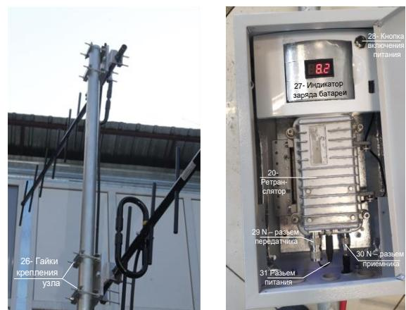
a) receiving antenna at the top and transmitting antenna at the bottom of the mast
