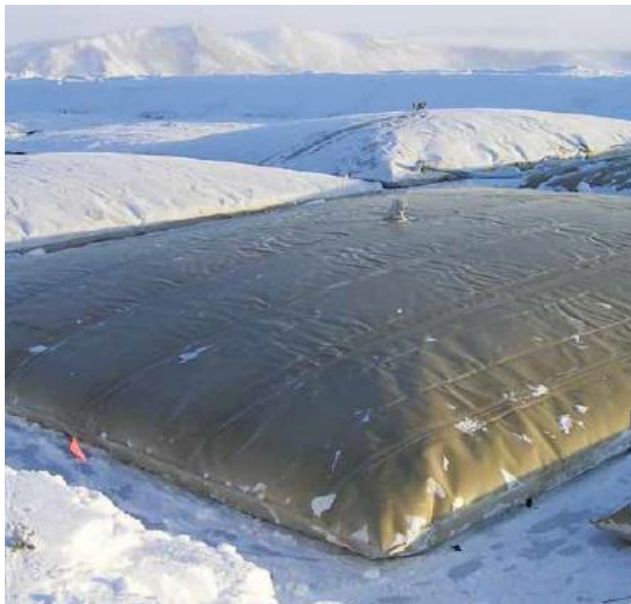
Figure 1 - Soft fuel storage tank
